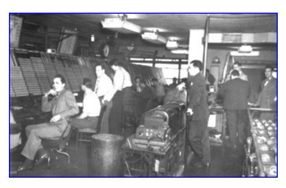
February 16, 1940 Station WSY CAA authority at LaGuardia Field operated the first overseas and foreign airways communication station (OFACS) with regular operations. It was capable of 2 way radio communications with aircraft flying the Atlantic Ocean.
